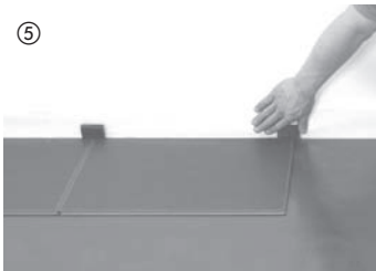
Starting in the left-hand corner of the room, align the boards of the first row with the tongue side parallel to the wall, and fix them in place with wall spacers or plastic spacers as you proceed (always keep an expansion gap of 10 - 15 mm (3/8" - 1/2") around perimeter).
