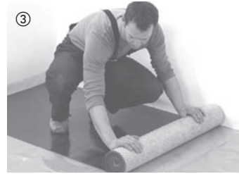
For sound insulation and to smooth out slight irregularities of the subfloor, unroll 2 mm thick Silent cork underlay. Do not overlap. Our range of accessories also offers alternative insulation underlays. Asphalt-bitumen felt is not suitable for sound insulation.
