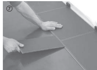
An easy trick to ensure a smooth interlocking of the Celenio boards at the short sides is to temporarily angle a leftover board piece lengthways into the two boards you want to click together.
