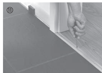
In doorways, mount a suitable moulding system to ensure the necessary expansion space. This also applies if the same floor is to be laid in the adjoining room. Leave an expansion space of approx. 5 mm between the board and the base of the moulding. As a rule, a fine saw must be used to cut a gap the thickness of a board in wooden door frames to allow Celenio to expand.
