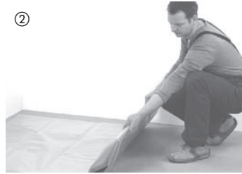
Always use 0,2 mm thick PE film overlapped by 30 cm as an underlayment when laying your HARO floor over concrete screed or cast plaster subfloors or over underfloor heating. Extend underlay up all walls. After having installed the skirtings cut underlay at the upper edge of the skirtings.
